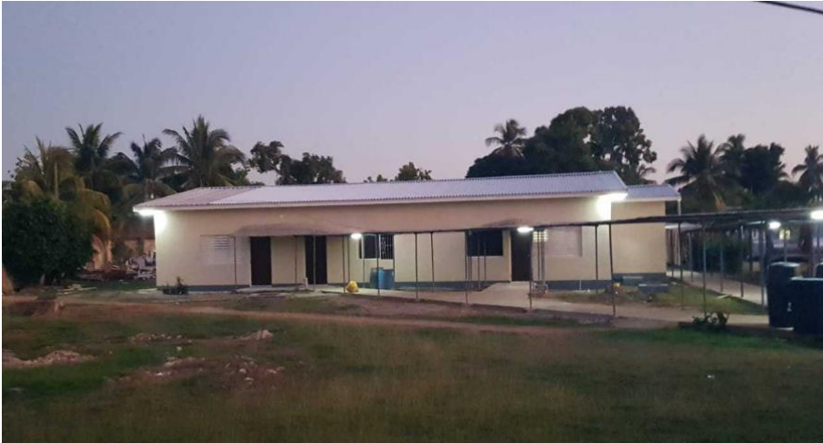
Renovation of New Location for Day-care Facility (In progress Pic # 1)
