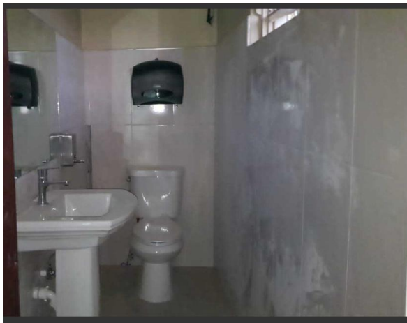
Renovation of New Location for Day-care Facility (In progress Pic # 2)
